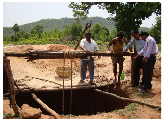
Ring well under construction at Brahmopanga, Kandhamal
